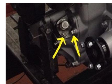
'Sealing 9' – Speedo drive/Gearbox end casing
